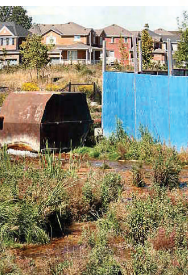
Sewer Construction discharge leaves brown metallic stain as it runs towards sensitive Rouge stream (September 2003).
