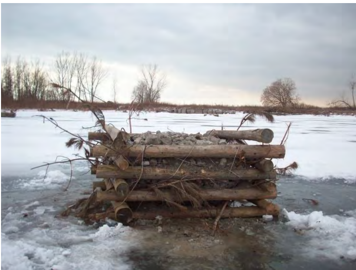
Figure 55: Log crib left on ice of Embayment A, March 2010. (TRCA 2010)
