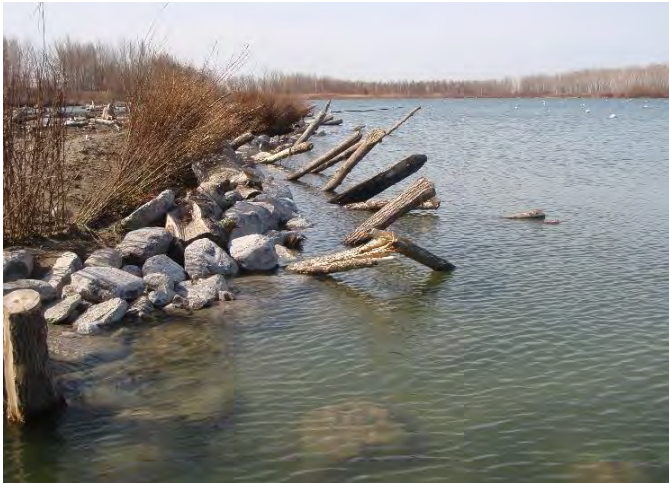
Figure 64: Live stakes, nearshore boulder shoal and anchored log fringe of the created wetland berm in Embayment C, South Shore. (TRCA 2011)
